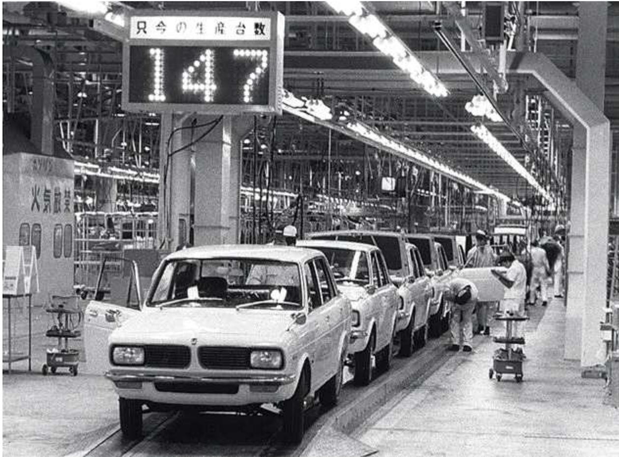
*The H1300 assembly line at Suzuka. The smoothness of production was the result of numerous efforts on behalf of the designers, engineers, and workers.*
